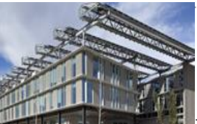
Cerdanyola del Vallès-Barcelona 5,700 m 2 SEM Electromechanical Systems. COM Communications. RF Actives
