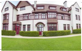
Las Arenas-Vizcaya 7,969 m 2 SEM Electromechanical Systems
